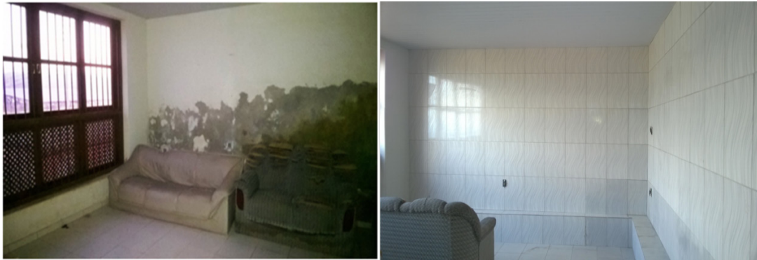
Figure 1: CCBP room 1 pre-reform and post-reform.
